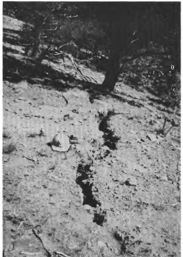
FIGURE 3.—Large open fissure associated with longwall mining in mountainous terrain near Raton, New Mexico. Such features can divert surface runoff, increasing landslide potential.
