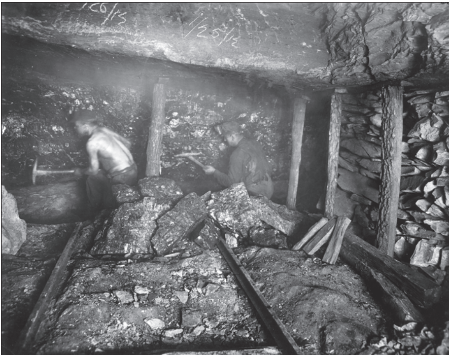
Figure 5 Photograph of mining at the face in an early longwall mine. Note the rock support on the right side of photograph. These mines operated from the 1870s to 1951 in fifteen counties. Most were located in the northern counties from Bureau through Will (fig. 2).
