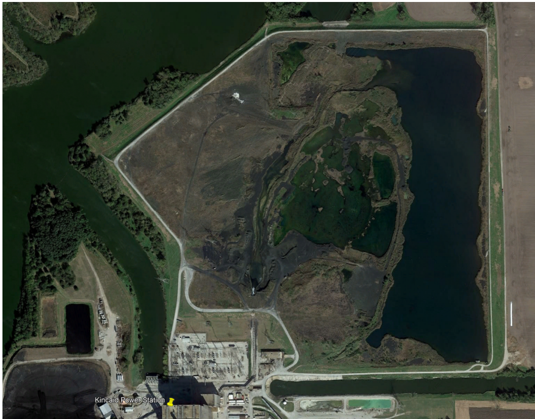
Figure 1 Vistra Kincaid CCR Pond
