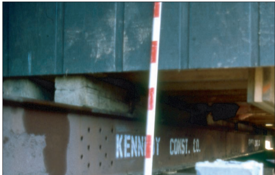
Figure 17 Concrete blocks of a crawl space have been removed to make room to jack the house to a level position. I-beams support the re-leveled house.
