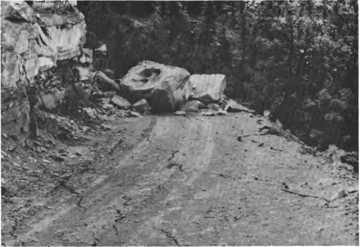
FIGURE 4.—Rockfalls and tension cracks produced during longwall coal mining near Raton, New Mexico.
