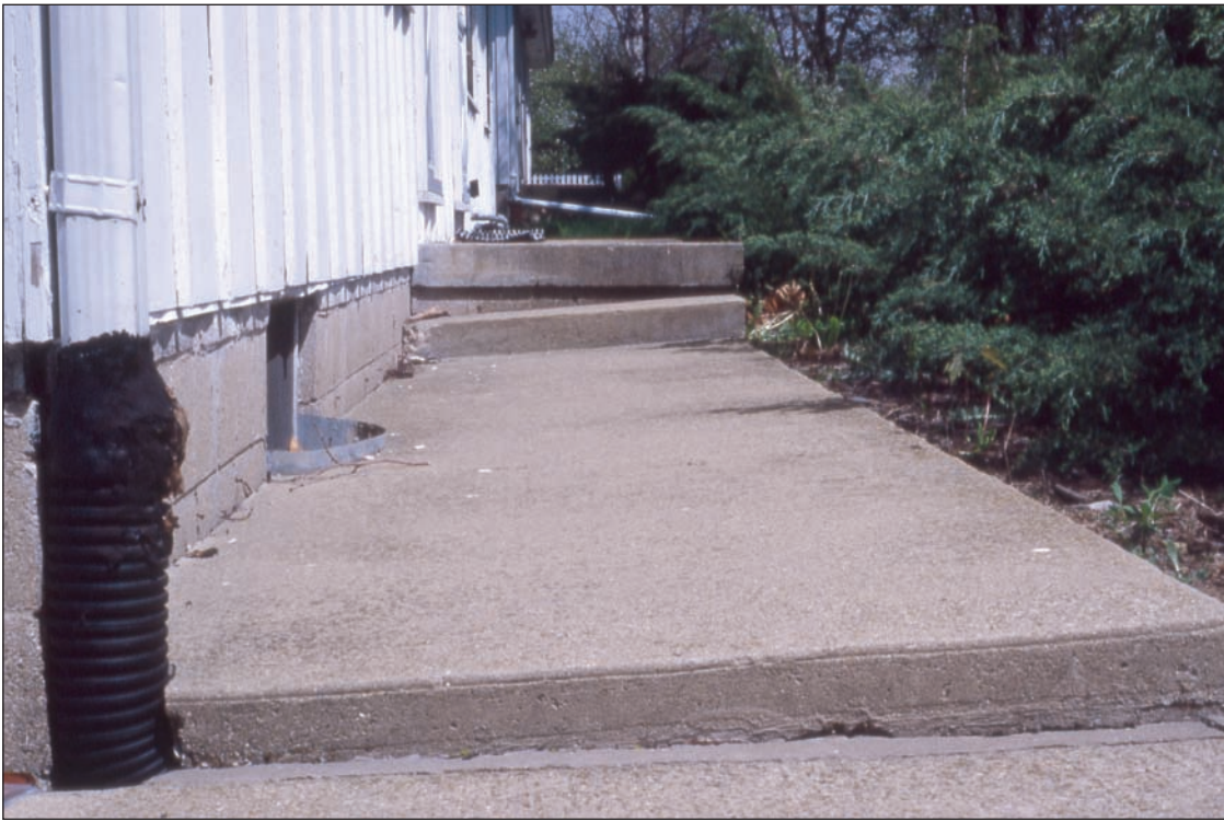
Figure 24 A moat-type depression along the foundation wall and lowered sidewalk and patio slabs caused by the kind of peripheral drainage system shown in figure 23.
